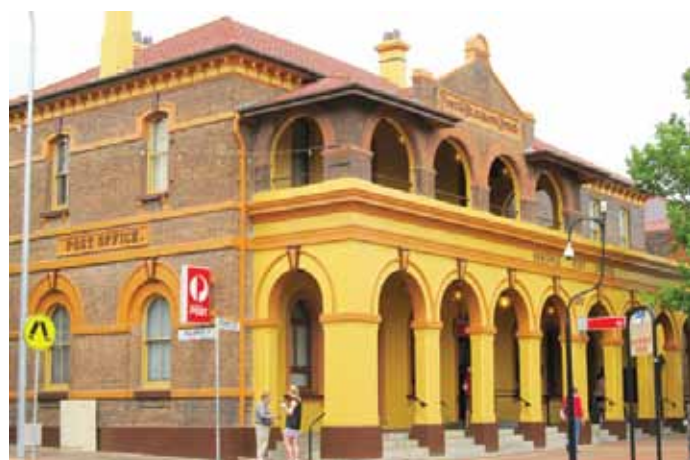
» ARMIDALE POST OFFICE , built in 1880, is unusual as it combines a Free Classical palazzo form with an attached stuccoed loggia.
